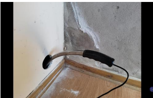
Overflate vegg - Veggflater 1
