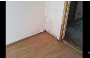
Overflate vegg - Veggflater 2
