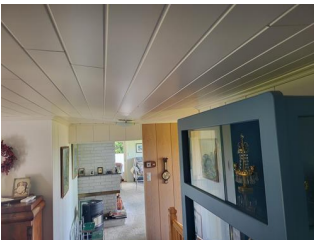
Overflate himling - Himling i gang
